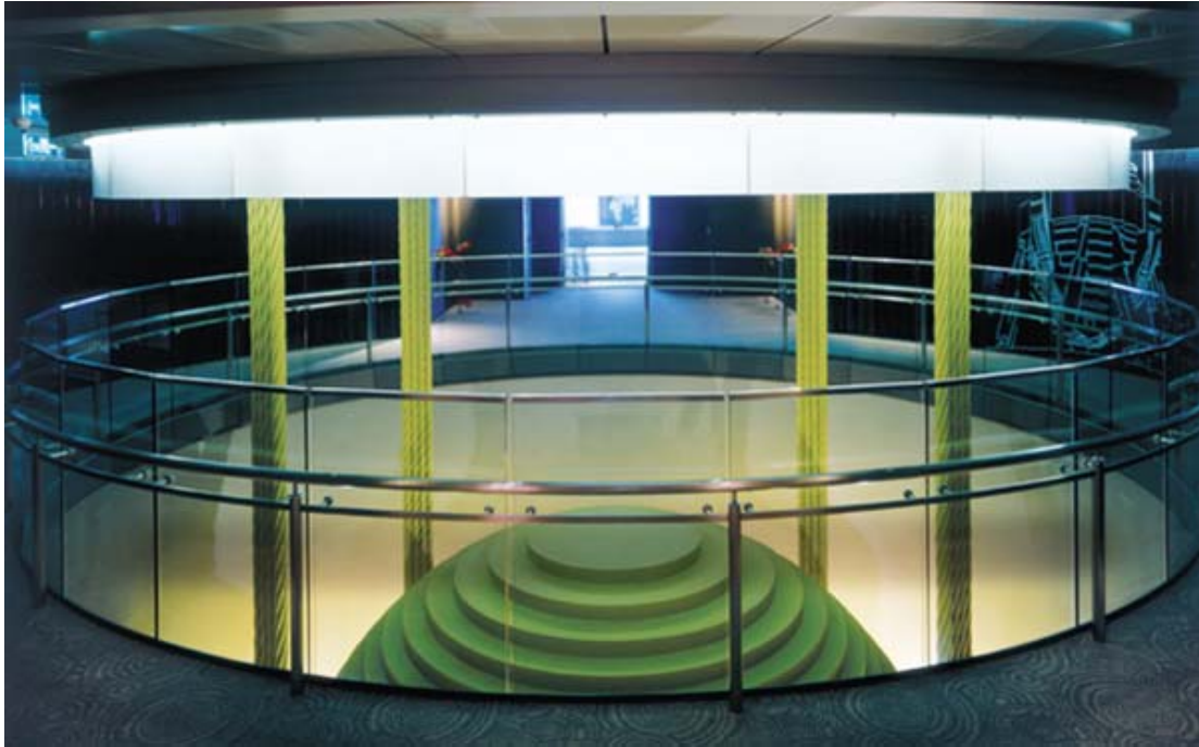
Pendular damper in the Taipei 101 Tower
